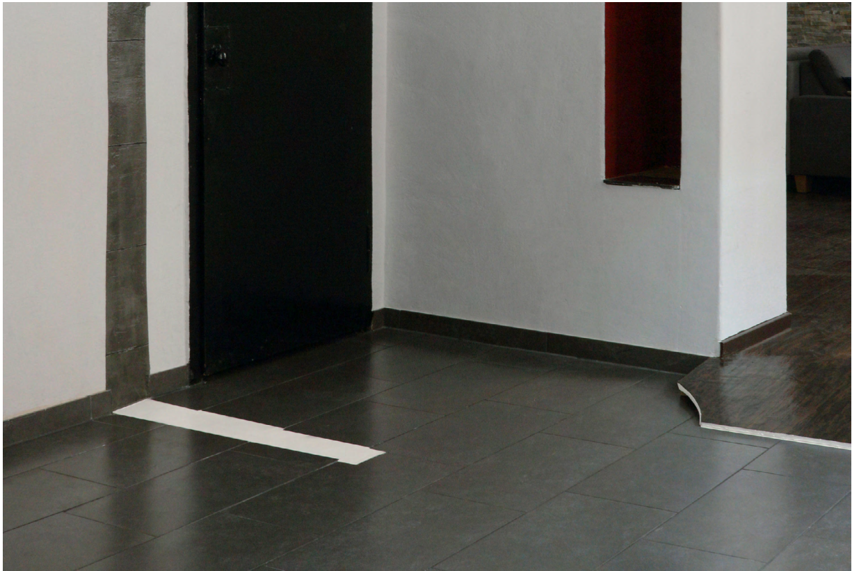
15 The demolition of a “wall of shame” made room for the wheelchair turning space required to gain eligibility for public funding.
