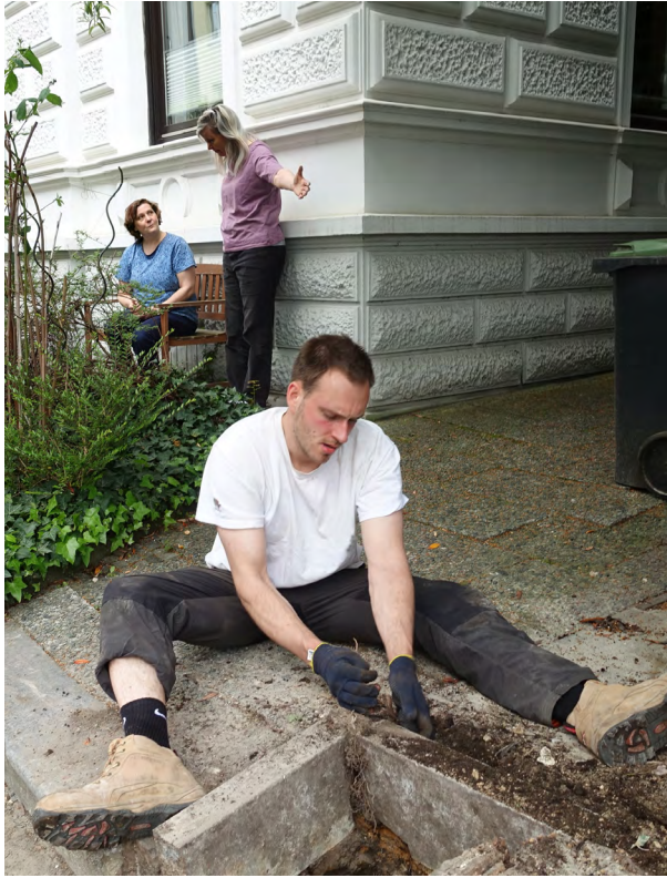
1 A student removes the roots of a dead tree that had affected the foundation of a brick pillar, leaving it in danger of collapsing. Authors' note: the faces of the women in the background have been anonymised using AI and image editing tools.
